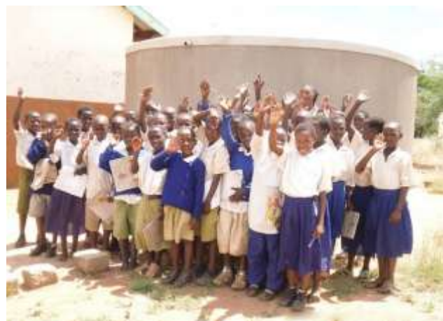
Children at Bugayambebele school in front of their new 30,000 litre rainwater harvesting tank that now provides a supply of clean drinking water.
